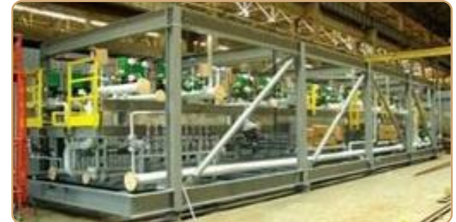
PSA and Burner Control Skid, Atyrau Refinery Reconstruction, Kazakhstan, AXSIA HOWMAR
