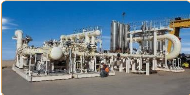
Rominserv Storage Tanks Farm Revamping, Romania, EMERSON-DANIEL
