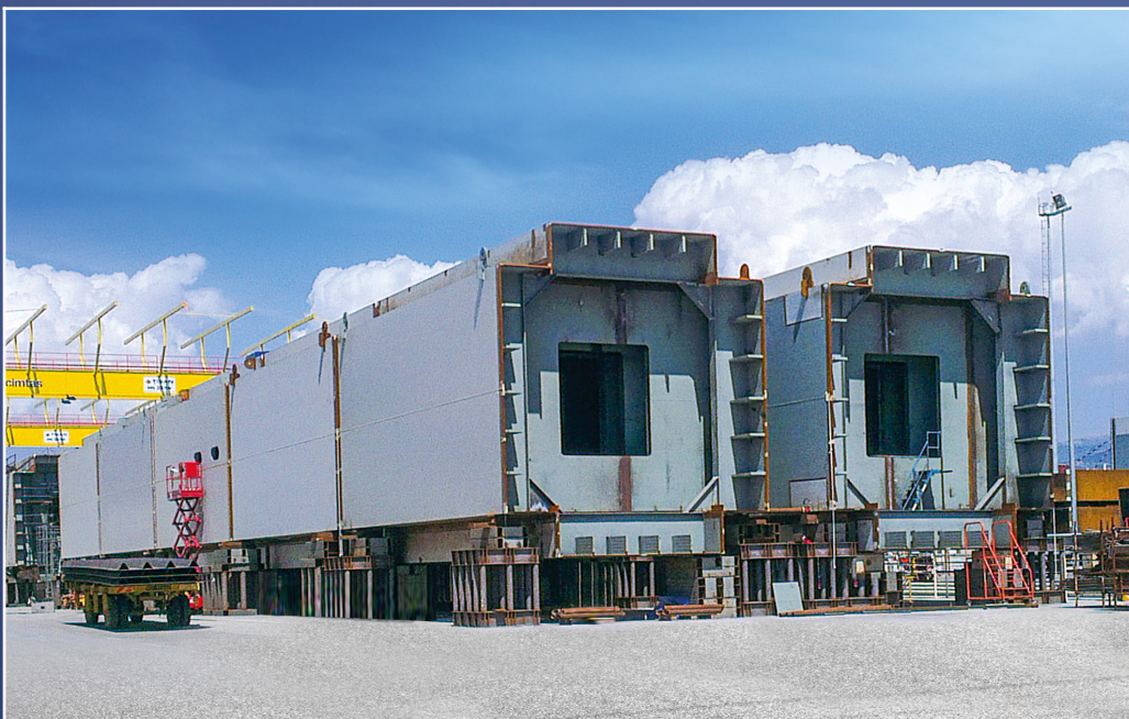
TOWER BLOCK TRIAL ASSEMBLY
