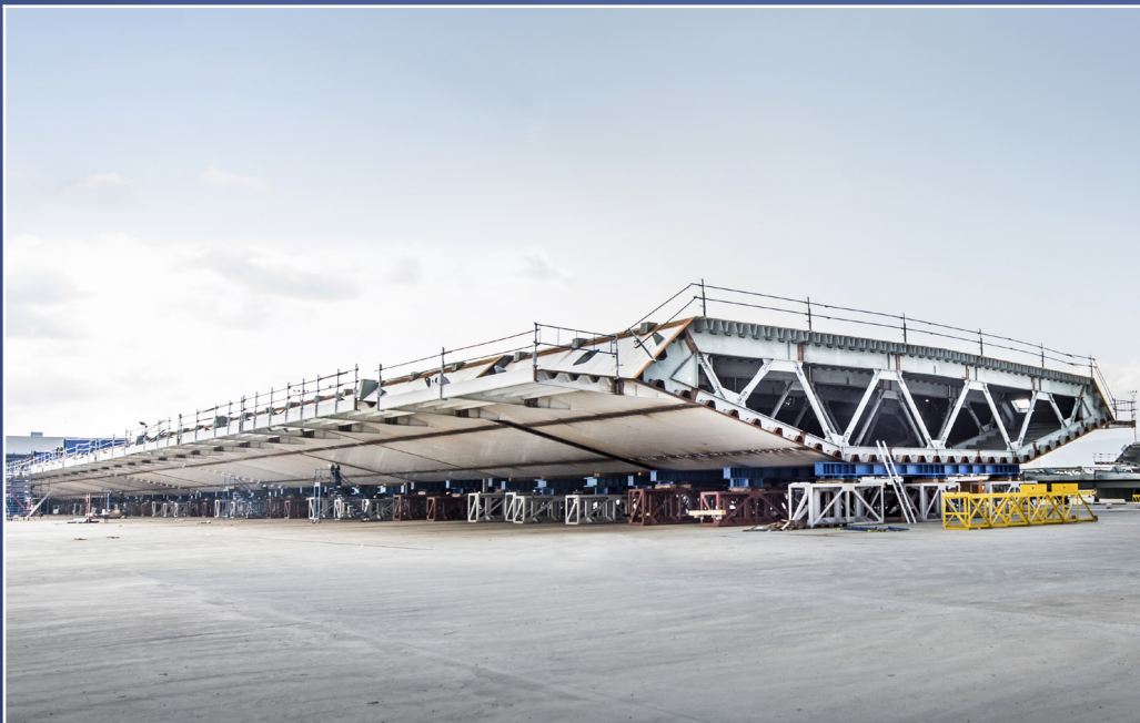
GIRDER BLOCK TRIAL ASSEMBLY
