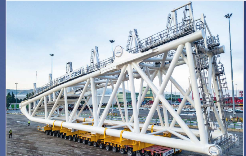
STINGER SECTION PROJECT
