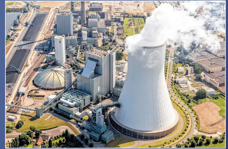
WALSUM COAL FIRED POWER PLANT
