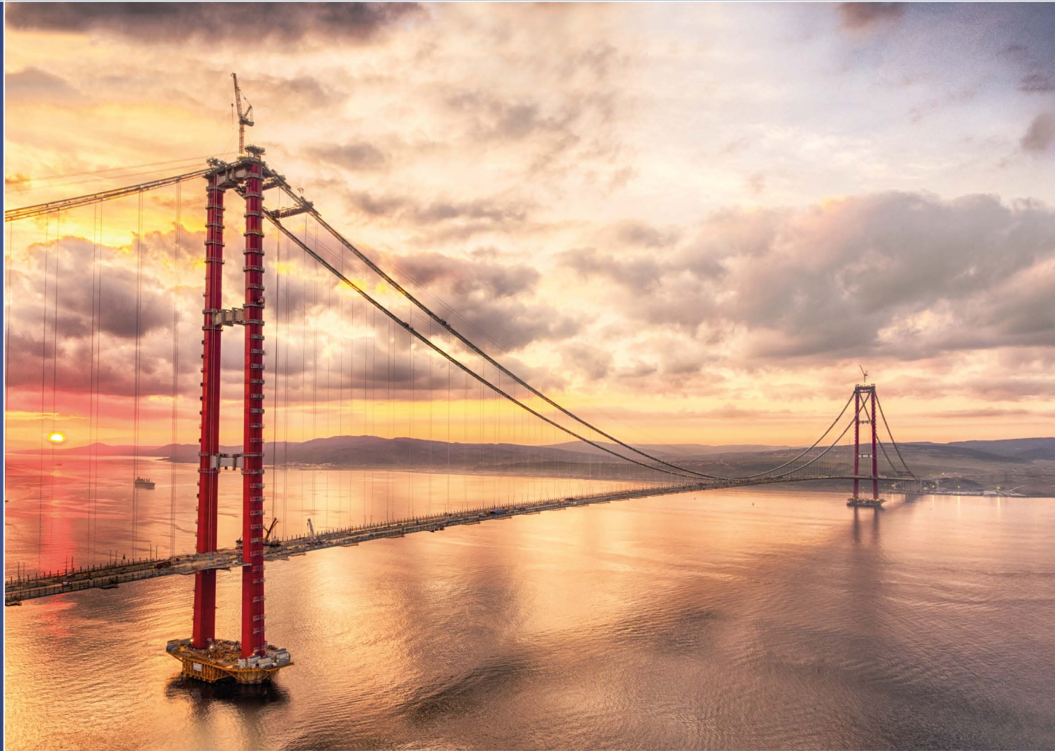
1915 ÇANAKKALE SUSPENSION BRIDGE The World's Longest Suspension Bridge
