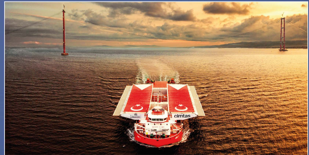
GIRDER BLOCK TRANSPORTATION
