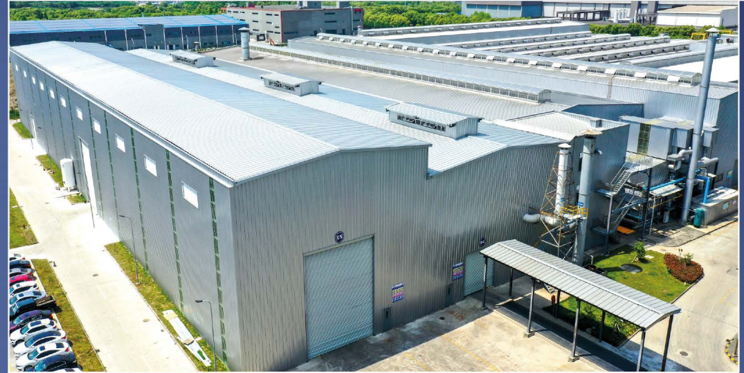
HIGH MODULE ASSEMBLY BAY
