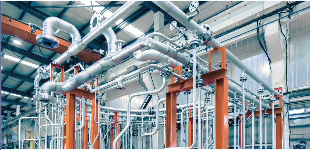
MITSUBISHI POWER AMERICA M501J JIG
