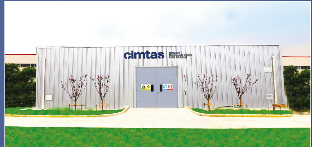
CHEMICAL STORAGE AREA CAPACITY: 40 ton
