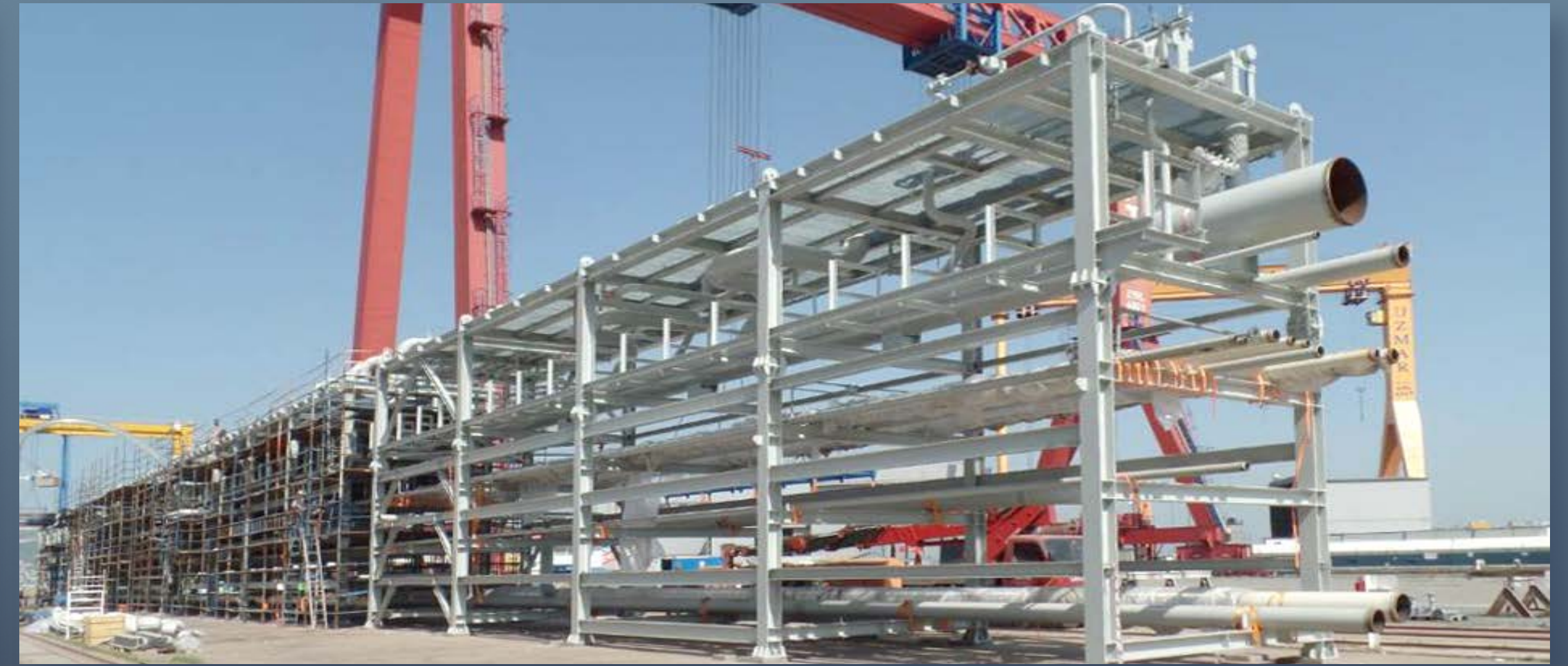
MODULE TRIAL ASSEMBLY
