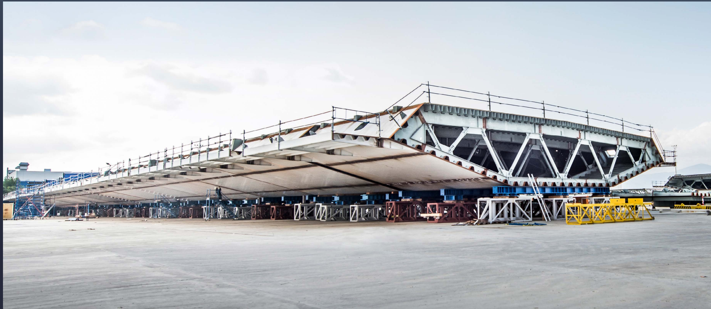
GIRDER BLOCK TRIAL ASSEMBLY
