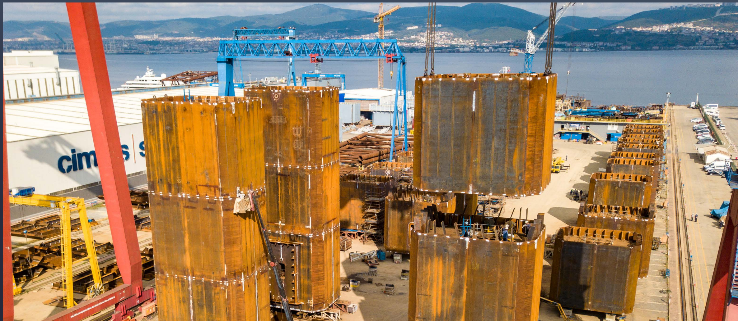
TOWER BLOCK TRIAL ASSEMBLY
