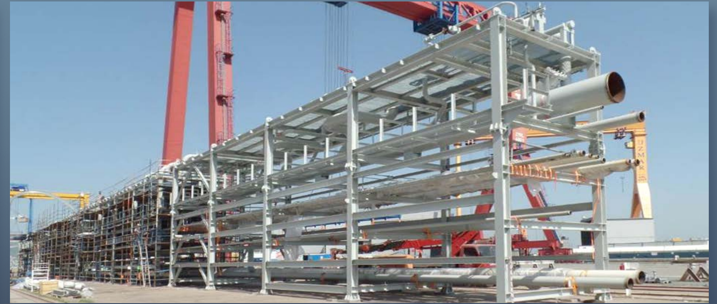
MODULE TRIAL ASSEMBLY
