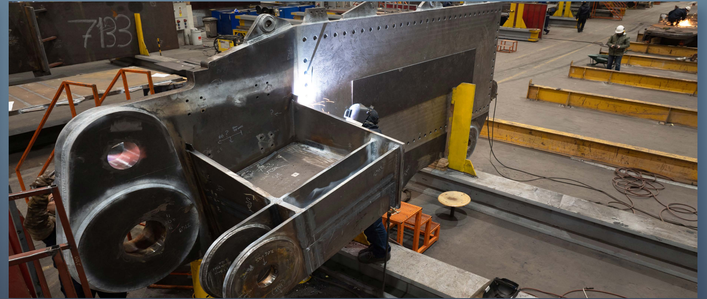
CAMP NOU STADIUM COMPRESSION RING FABRICATION
